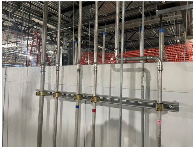
Food Processing Facility – StainlessPress® Applied to Hot & Cold Water Returns As Well As Chemical Processing
